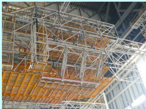
Tail dock with direct Auxiliary Power Unit access design
