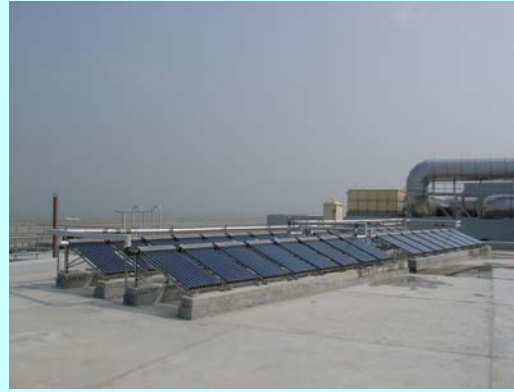
New Solar water heaters installed at Hangar 3 in 2009
